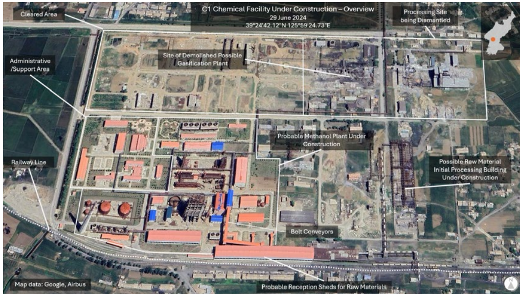
Figure 18: Overview of the C1 Chemical Facility under construction
