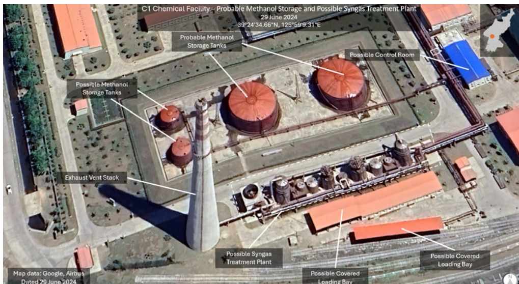
Figure 23: Probable methanol storage and possible syngas treatment plant
