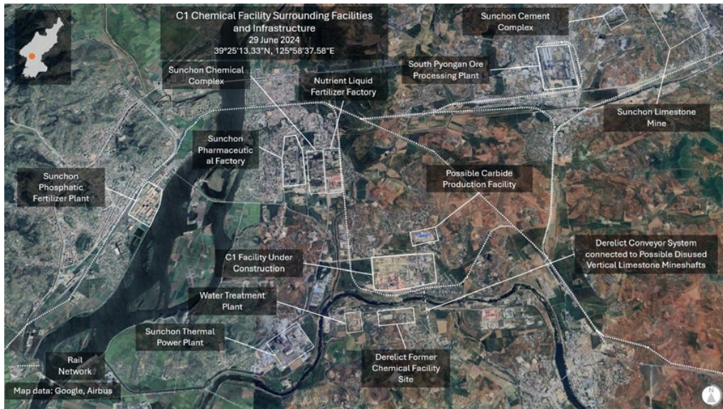
Figure 19: Overview of surrounding facilities and infrastructure of the Sunchon C1 Chemical Facility
