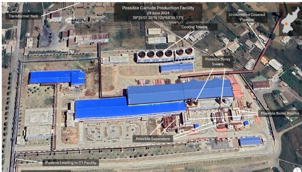
Figure 26: Possible carbide production facility
