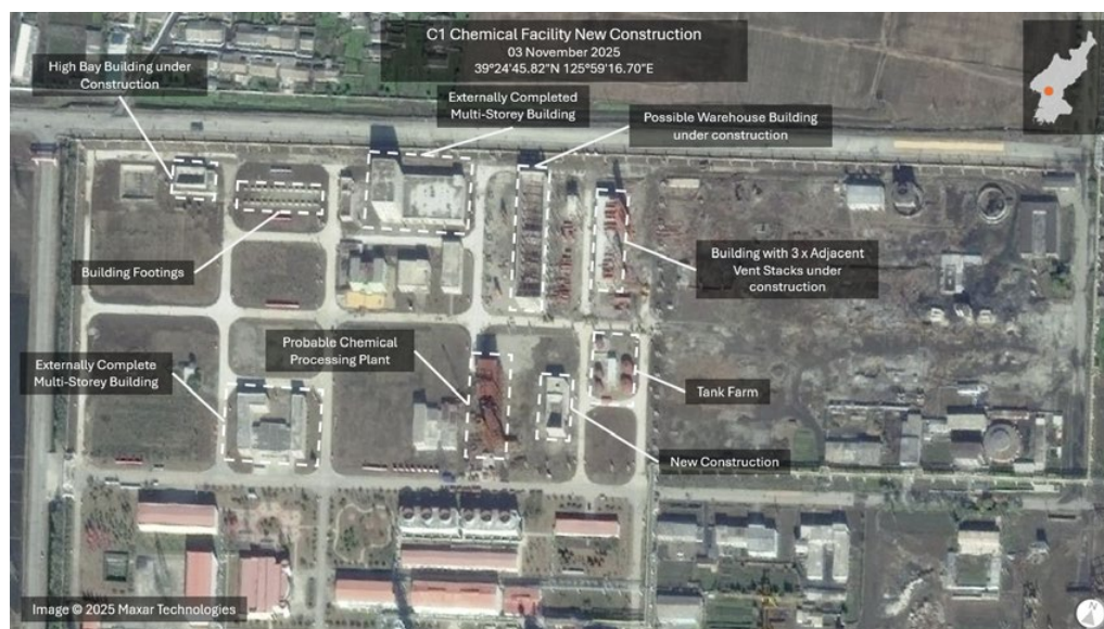
Figure 27: Cleared area under construction at the C1 Plant.
